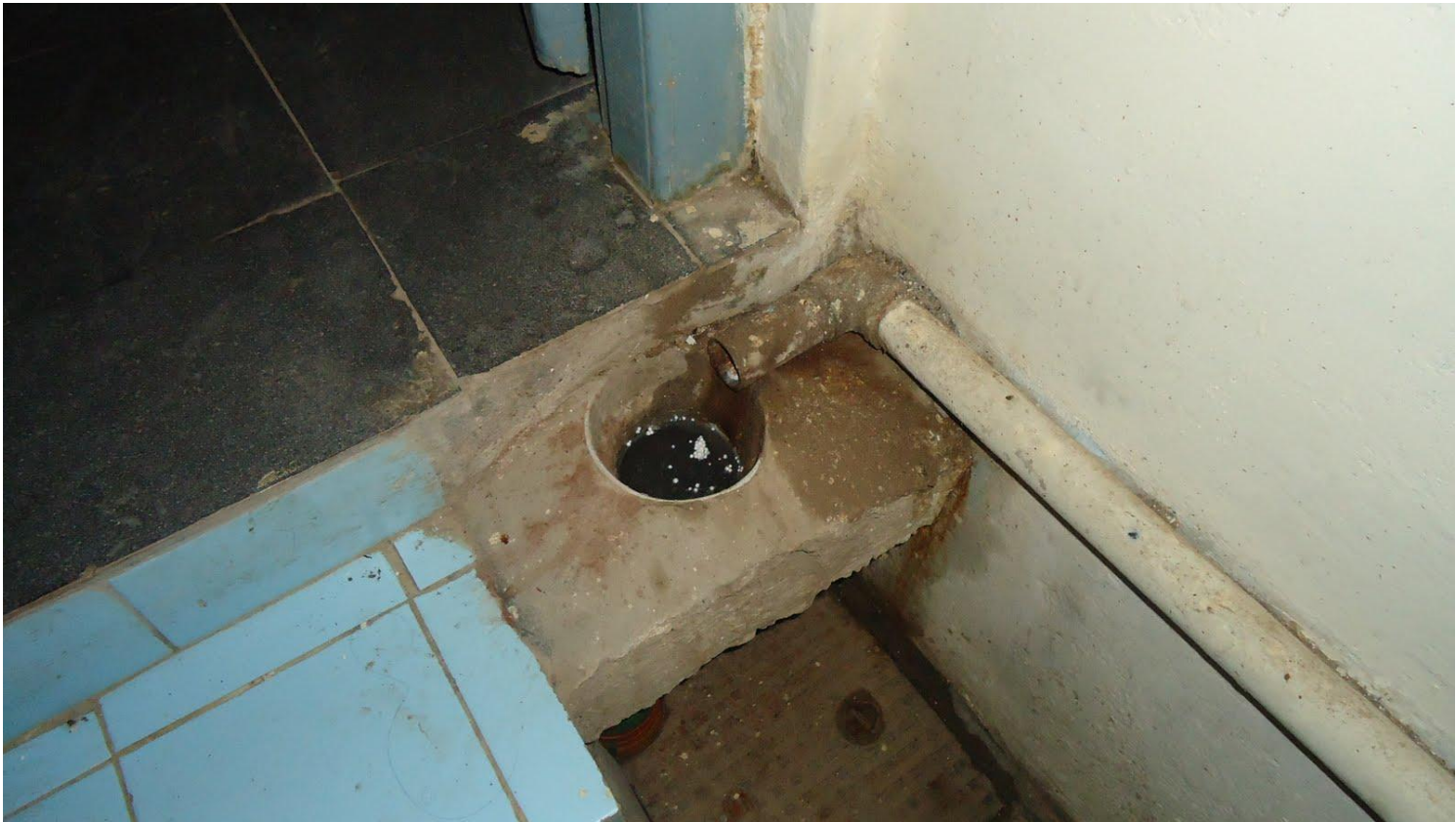
Newly constructed open drainage after rise in road level
