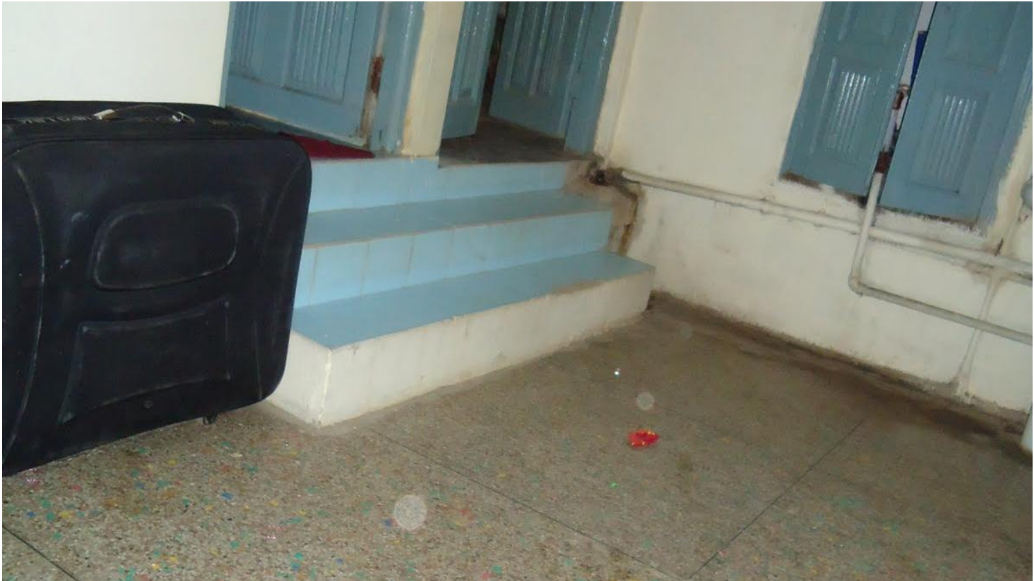
Newly constructed stairs after rise in road level
